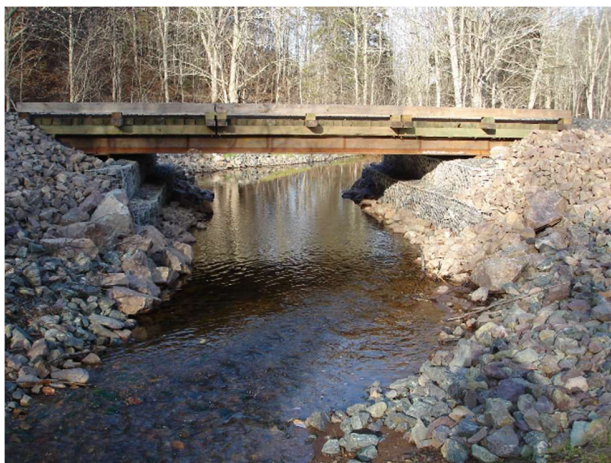
New bridge installation, Paul MacDonald, PHP
